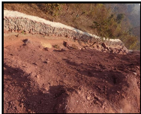
Retaining wall provided at the toe end of the dump
