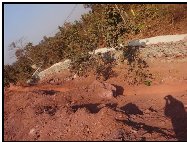
Retaining wall provided at the toe end of the dump
